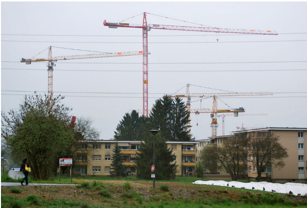
Fig. 2 Construction cranes rise above existing housing stock
