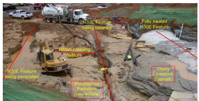
Fig. 5 Cleaning of N30E features
