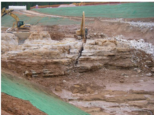
Fig. 2 Irregular packstone surface detected in seismic refraction survey
