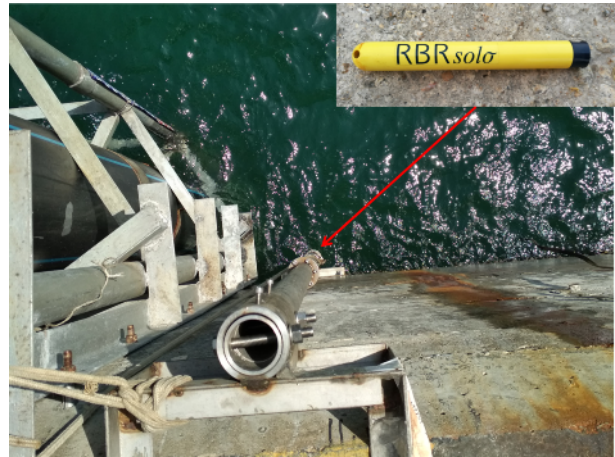
Fig. 5. RBR tide gauge. The tide gauge is fixed by stainless steel tube to ensure the vertical of tide gauge.
