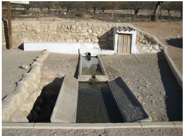
Fig. 1 Drinking trough and washing space at the end of the qanat's pithead in Fuente Grande (Los Vélez, Almería)
