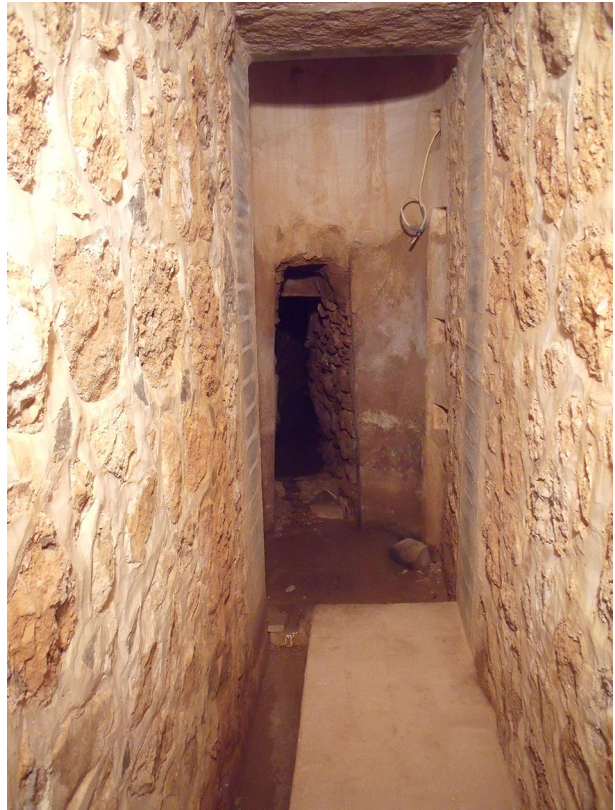
Fig. 8 Interior view of the ganat of Casa Herrera (Jumilla), in the foreground rehabilitated part; in the background, the original part of the gallery
