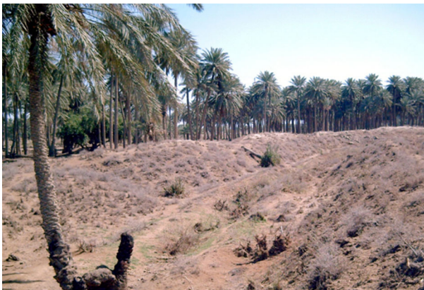
Fig. 11 Canal located close to the Hilla branch in the western plains; this was dug around 1935 by hand shovels and shows how large amount of sediments accumulate alongside the canal (Jaafar Jotheri)
