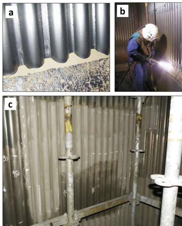
Fig. 12 Protective coatings deposited by thermal spray in fluidized bed power boiler a after 1 year of operation, b coating regenerating process above the lining and c regenerated coating after 9 years of service [11]
