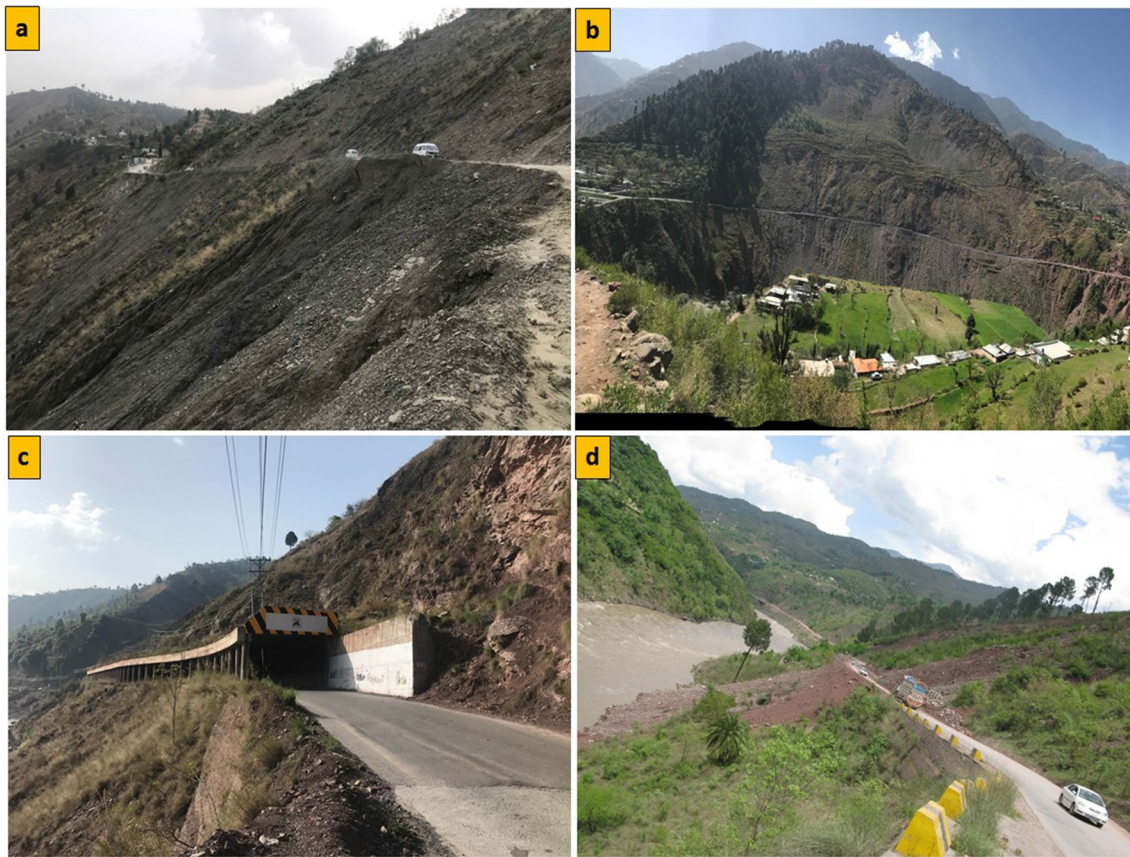
Fig. 3 Field photographs of landslide events along the study area road corridors: a Lohargali landslide along Neelum road, b Panjgaran landslide along Neelum road, c Subri landslide along Jhelum Valley road, d Rara landslide along Kohala road
