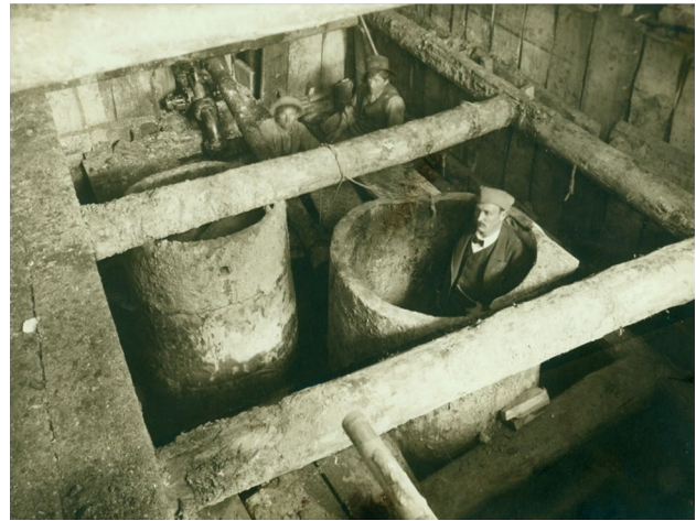
Fig. 11 Excavated wooden tree trunks Nr.2 and Nr. 1 of original Bronze Age spring capture of St. Moritz Mauritius mineral spring in 1907 (Photo under copyright, by Permission of Museum, St. Moritz, documentation section, 8.4.2022)
