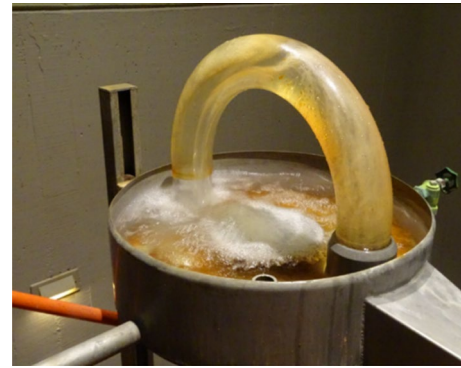
Fig. 13 Original Mauritius mineral spring capture outflow fountain with installed inner glass tube bow
