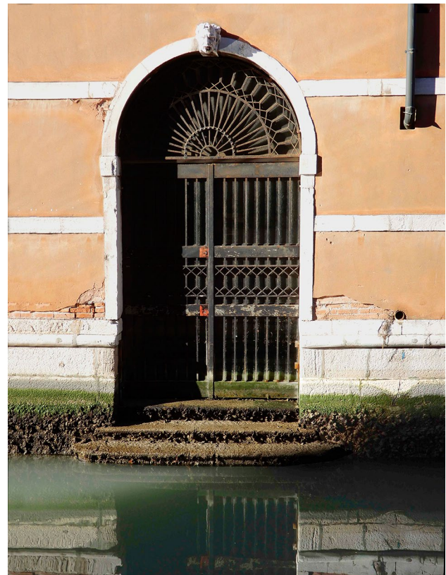
Fig. 3 At high tides, this sea stair is fully submerged. All steps are colonized by algae and shells. Nowadays this stair is totally impractical. The upper front of green algae is the level currently reached by sea water (normal tides and small waves). Picture taken at low tide
