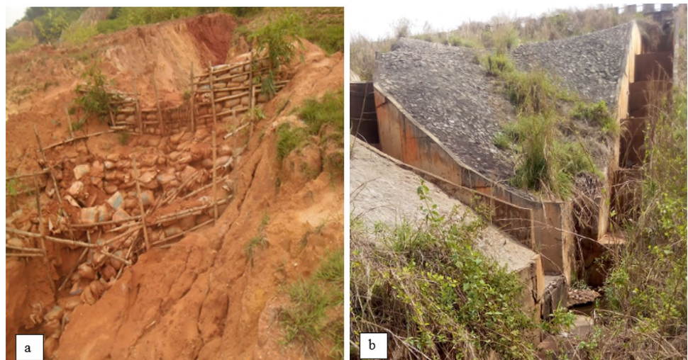
Fig. 1 Different technical methods used in the study area to check erosion: a sand bags (Igwe and Una 2019), b runoff breakers
