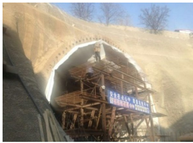
Fig. 1 Caomaoshan Tunnel entrance area
