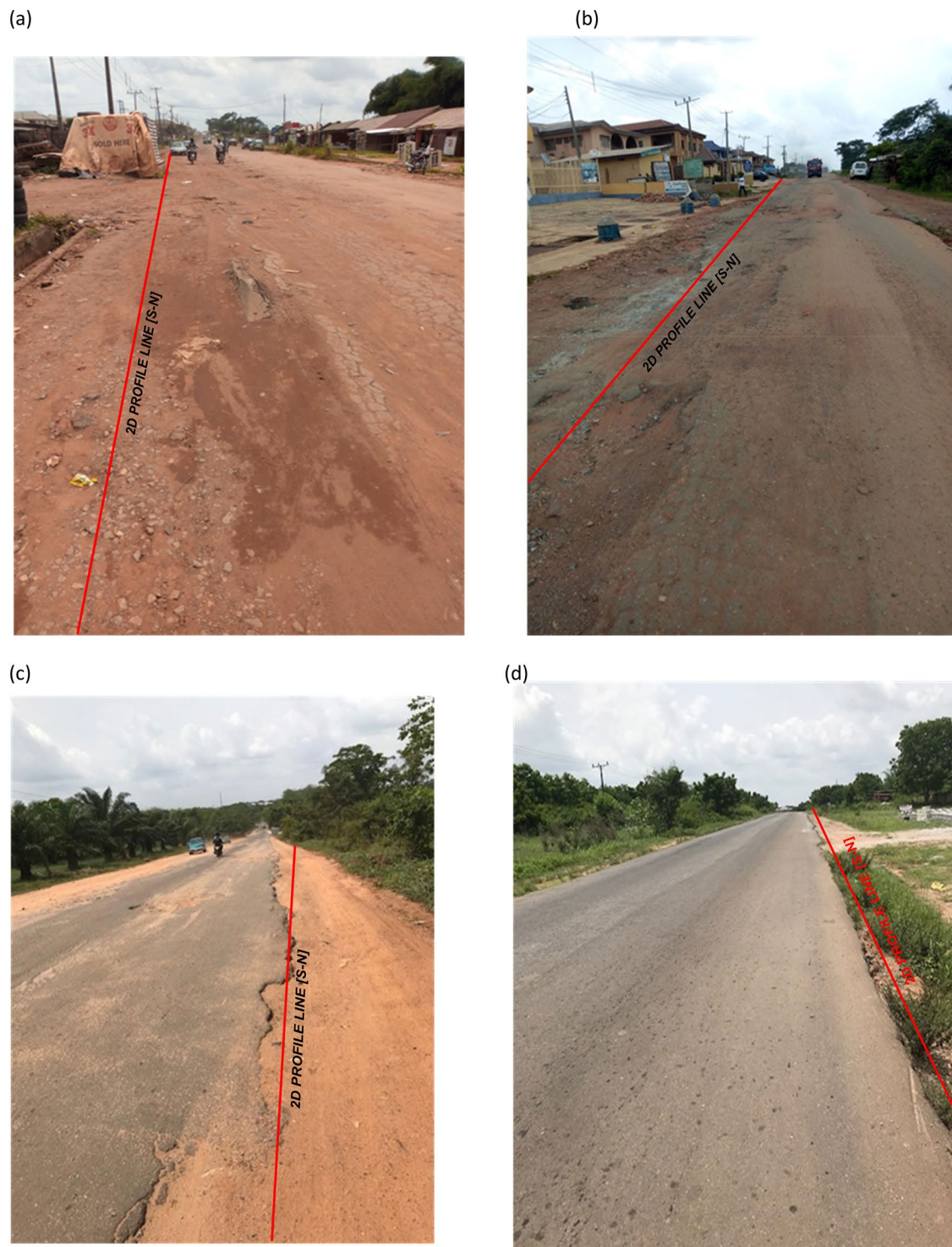
Fig. 1 Photo showing the state of the road. a Bad portion, b poor portion, c fair portion while d good portion of the road
