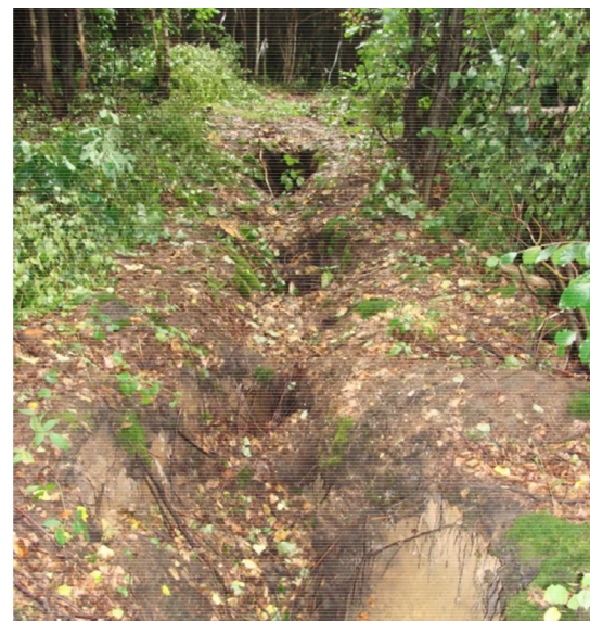
Fig. 2 General view of the series of sinkholes (author M. Gasz)
