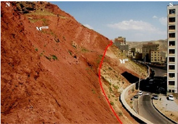
Fig. 6 Tower construction in the vicinity of Tabriz fault and on unstable geological formations
