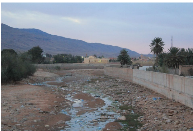
Fig. 11 Retaining walls in wadi Breidj
