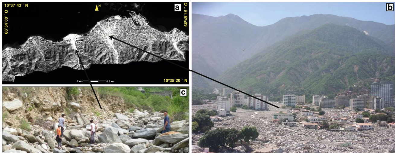
Fig. 1 Overview of deposits and effects of December 1999 debris flow event in Venezuela's Vargas state: a deposits (white color) of the event on the alluvial fans (from left to right) Macuto, Punta El Cojo, Camurí Chiquito, Punta El Caribe and Punta Cerro Grande, b impact of debris flows on the population (Los Corales sector) and c debris
