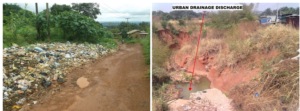
Fig. 3 Photographs of indiscriminate dumpsites and urban effluents discharge
