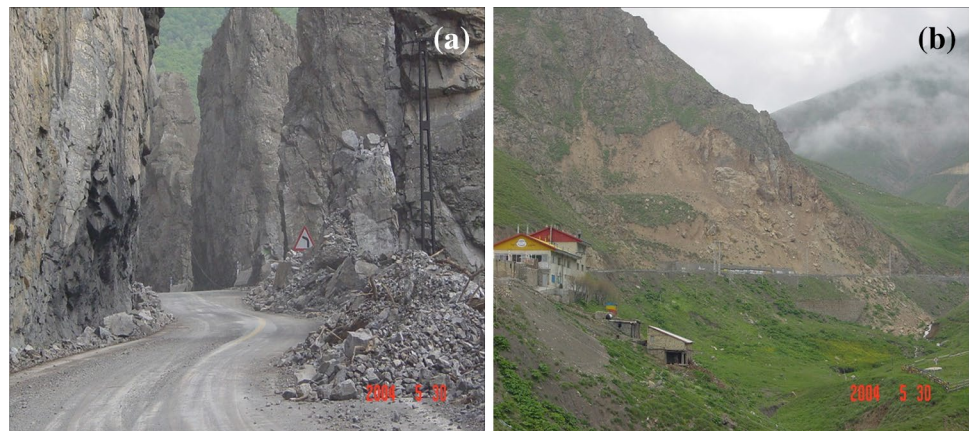
Fig. 6 Rockfalls triggered by the Firooz Abad-Kojour earthquake of 2004 within the study area: a falling zone in Chalus road, 12 km from Baladeh three ways to Chalus; b blockage of some parts of Chalus road due to rockfalls in 14 Km of Baladeh three ways to Karaj
