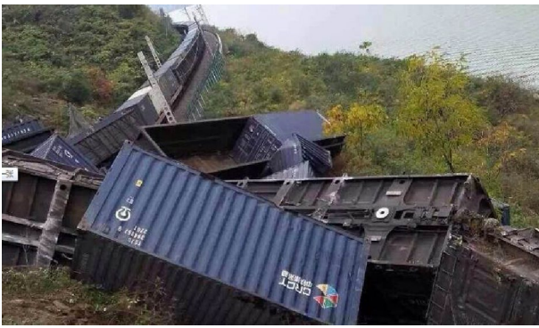
Fig. 1 Train derailment caused by a landslide () Cited from the network
