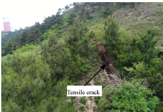
Fig. 19 Tensile crack around main shaft area
