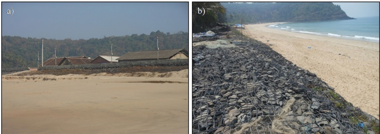
Fig. 9 Seawalls near a northern and b southern headland
