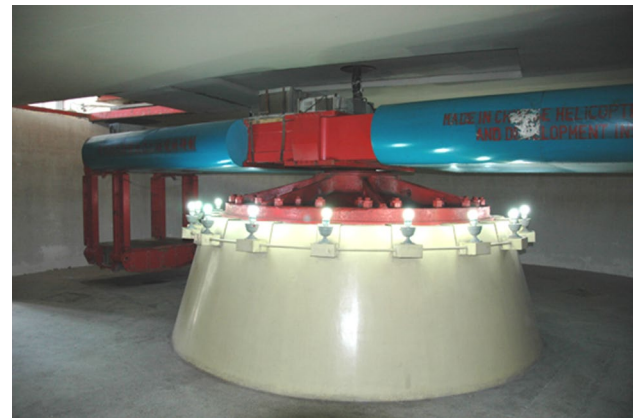
Fig. 2 Geotechnical centrifuge (NH-400 gt)
