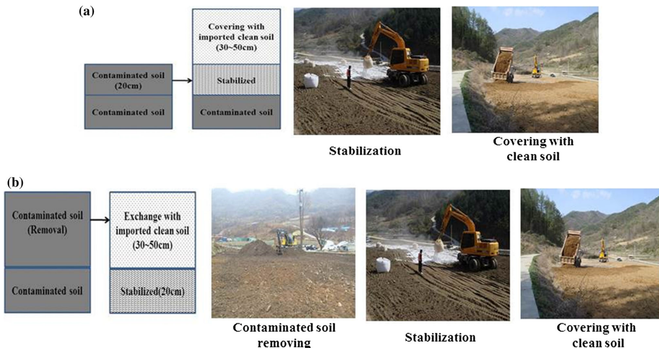
Fig. 1 A schematic diagram of soil reclamation methods for agricultural applications. a Stabilization and covering, b exchanging and covering
