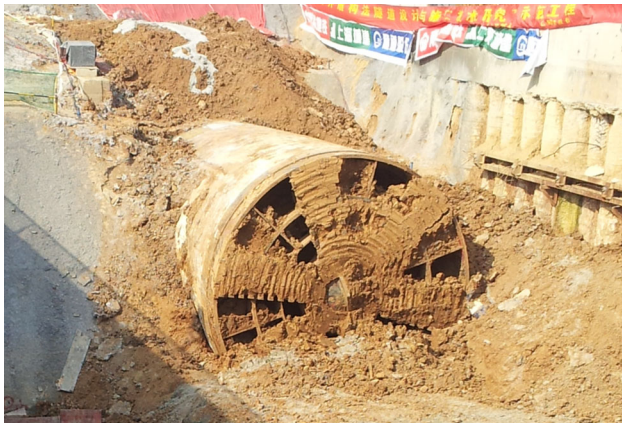
Fig. 13 Photograph of the URUP TBM during receiving on the ground surface
