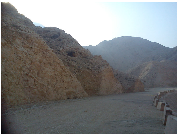
Fig. 6 A view of the discontinuous rock slope
