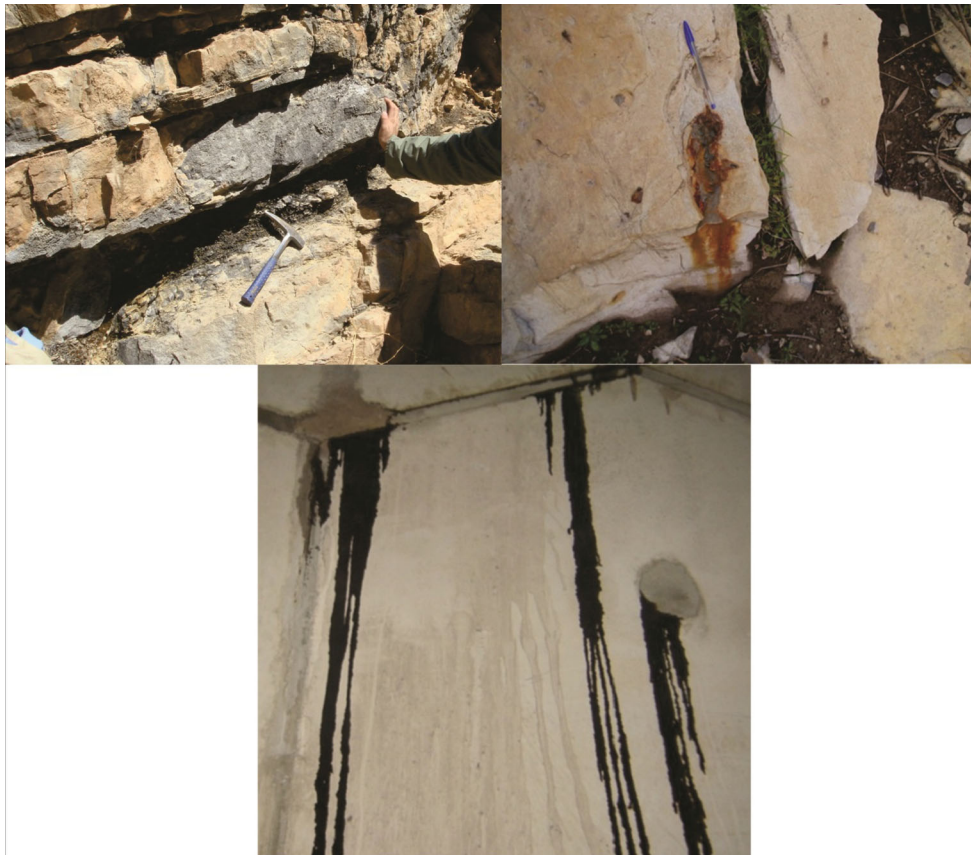
Fig. 7 Interlayer of shale between limestones in the Aspar anticline, seepage hydrocarbons materials into the tunnel in Pabdeh and Gurpi formations and Pyrite (sulfur balls) decomposition at surface (limonite)
