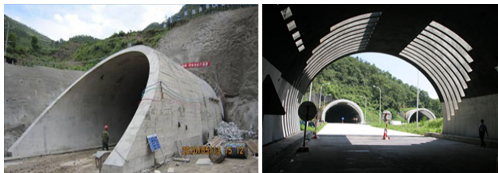
Fig. 17 The bamboo-truncating portal and ring frame tunnel portal
