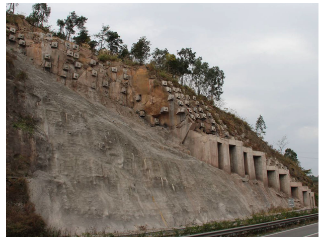
Fig. 15 Photograph of rock slope 2 years after stabilization
