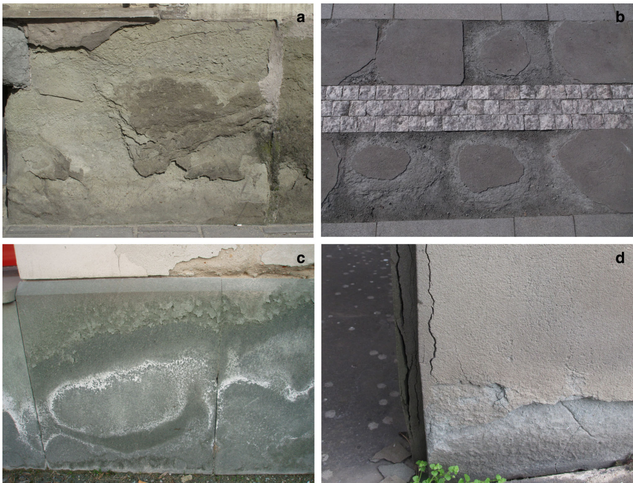
Fig. 5 Illustrative examples of Godula sandstone deterioration in buildings. a Blistering and crust formation on surface of sandstone block in the base of building (Jiří Myron Theatre in Ostrava built in 1892–1893; photograph taken in 2016). b Demonstration of extreme exfoliation of Godula sandstones after only ca 10 years of exposition in exterior (pavement at the entrance to the Ostrava–Svinov railway
