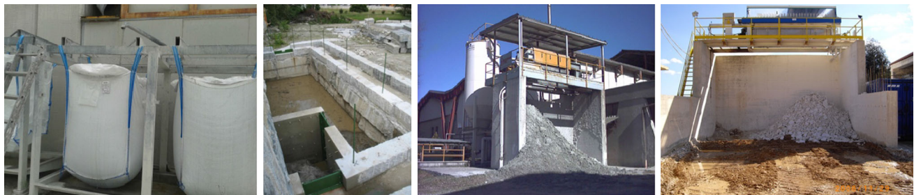
Fig. 2 Sludge treatment: big bag (a); settling basins/tanks (b); filter-press SS (c); filter-press CS (d)
