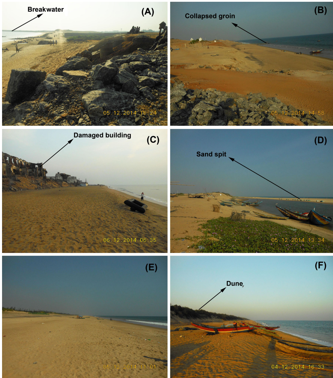
Fig. 9 Field photograph showing major locations along Ganjam coast. a Highly eroding Aryapalli beach located on the northern side of Gopalpur port, b partially collapsed groins in Aryapalli, c Gopalpur tourist beach, arrow indicate the collapsed buildings due to past
