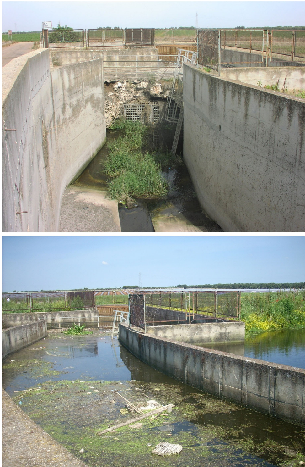
Fig. 5 Water levels in LB1 at Vora Colucce water sink. Above low water level during dry season (picture taken September 9, 2007); below high water level and surrounding flooding during wet season (picture taken April 4, 2010)
