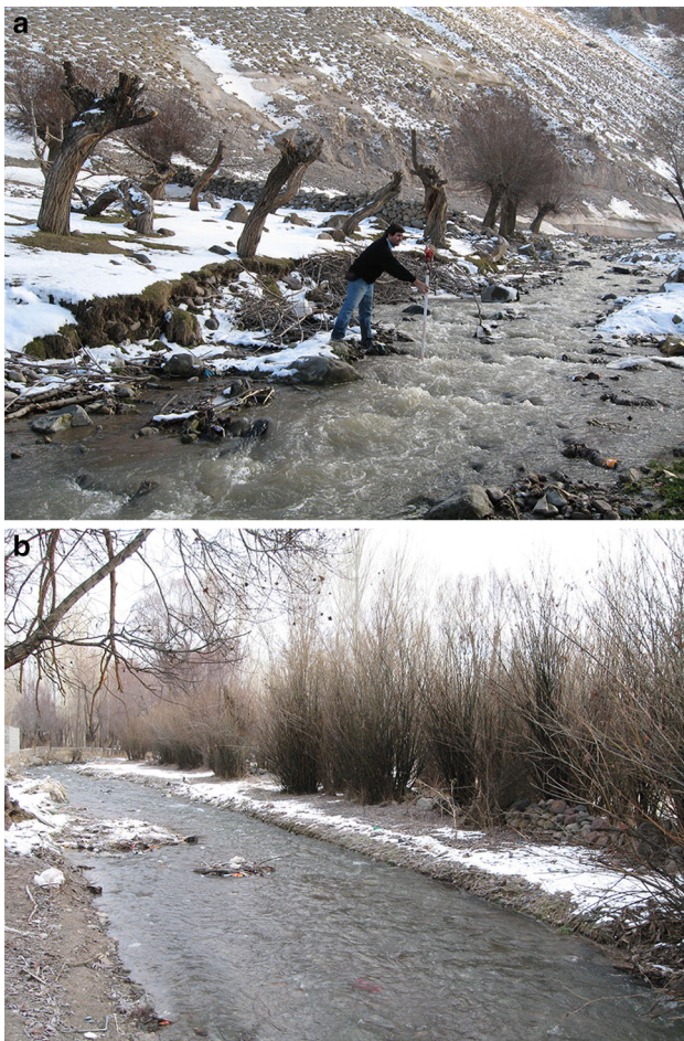
Fig. 2 Channel morphology of the Lighvan River. a upstream reach near Section 4; b downstream reach near Section 12
