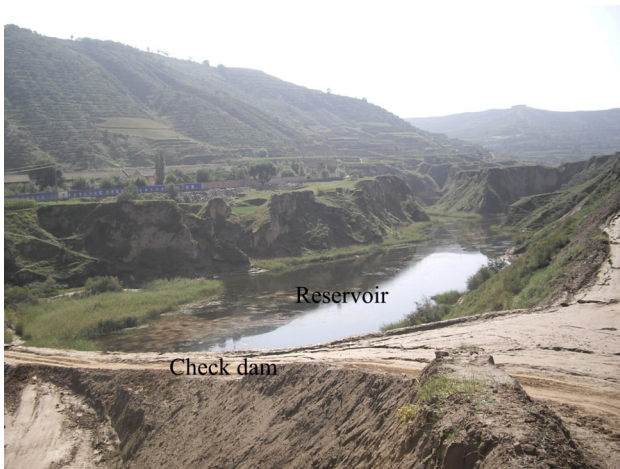
Fig. 8 A constructed dam system greatly reduced soil and water loss from the catchment (photo from 2010)
