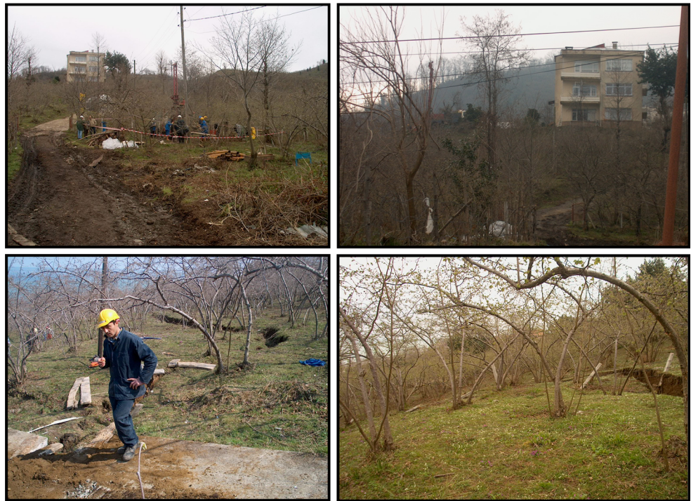
Fig. 4 Photographs of the Aksu landslide area. Top photos the landslide area looking SSE. Bottom photos the scarp of the landslide looking NE. Due to dense vegetation, the entire outline of the landslide cannot be observed in the photos
