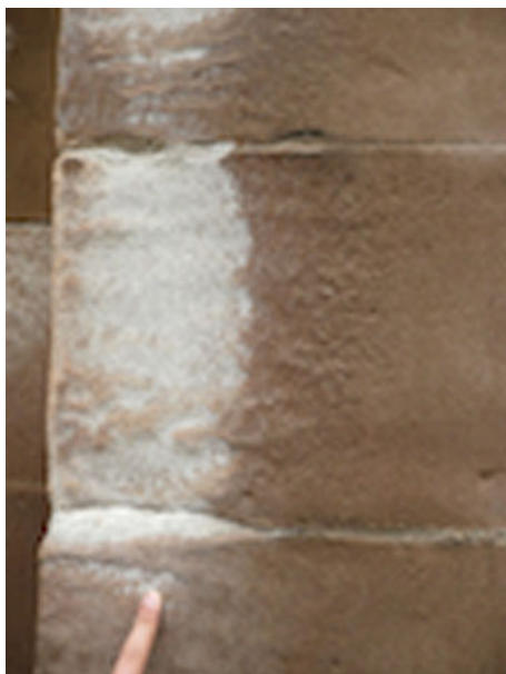
Fig. 1 A ‘traditional’ view of salt weathering damage, where frequent wetting and drying cycles bring about granular disaggregation on the surface
