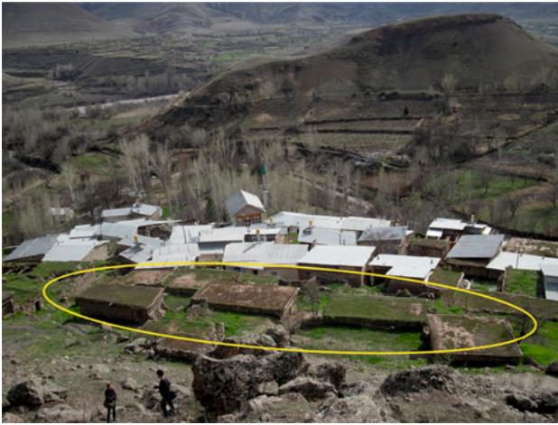
Fig. 11 Houses destroyed during the earlier rock fall
