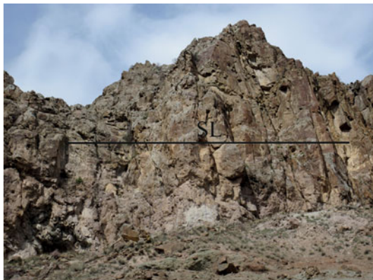
Fig. 4 Views from a scan line survey
