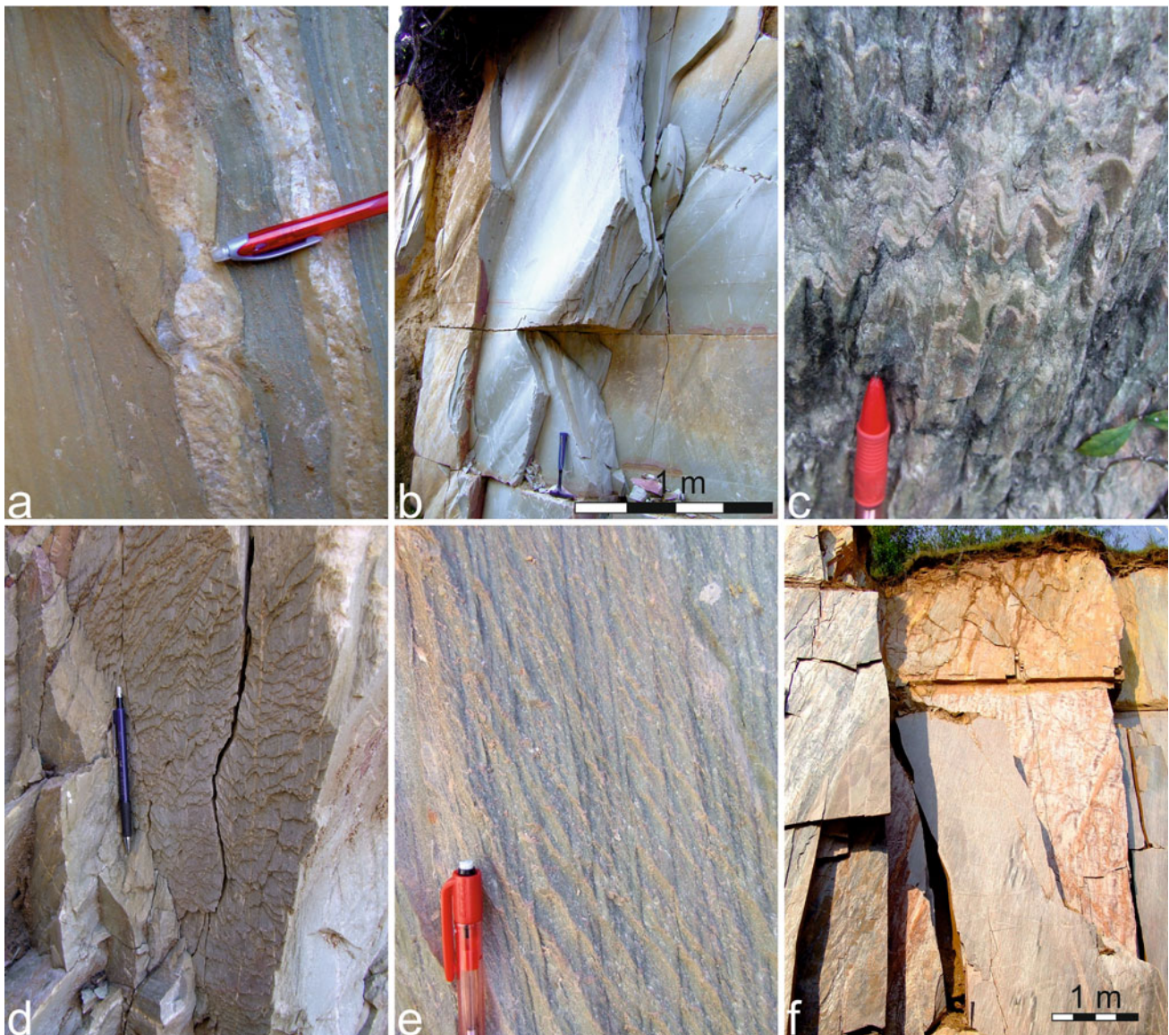
Fig. 17 Structural elements negatively affecting the dolomitic slate deposits in Uruguay. a Carbonate boudins with quartz necks. b Foliation in slate showing large amplitudes and very frequent kink bands. c Highly folded slate. d Scales develop where S_{0-1} and S_2
