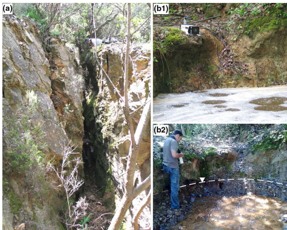
Fig. 3 a Esquerda de l'Infern (see person at the bottom for scale), an open crack formed by gravitational deformation of the mountain slope induced by recent coseismic activity on the Amer fault. According to historical data, this was the site where gas emanations took place during the 1427 seismic crisis. Triggered by the earthquakes, endogene gases either flowing out from the Amer fault along gravitational failure planes. Gas measurements recorded on June 17,
