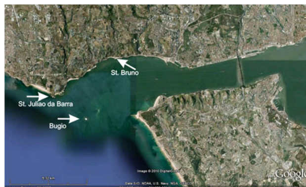
Fig. 1 Satellite map of Lisbon Harbour with the location of the three fortification monuments under study
