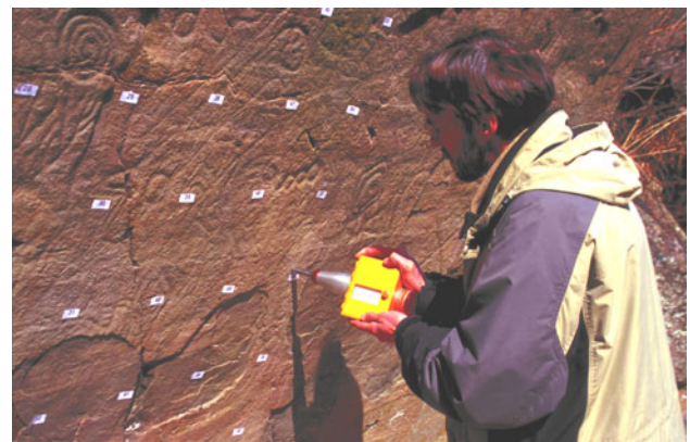
Fig. 6 Rebound hardness measurements with Schmidt hammer
