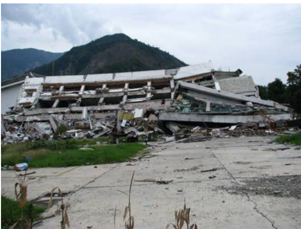
Fig. 2 Building damages at Beichuan Municipal Office
