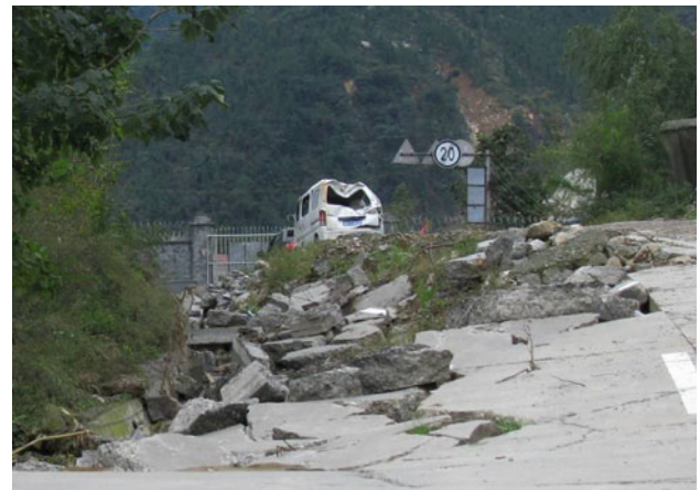
Fig. 3 Example of earthquake surface ruptures
