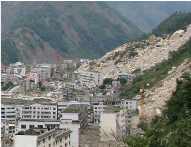
Fig. 4 Xinbei Middle School landslide at the new town in Beichuan
