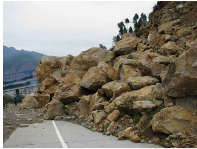
Fig. 5 Rockfalls on the road from Renjiaping to the old town in Beichuan
