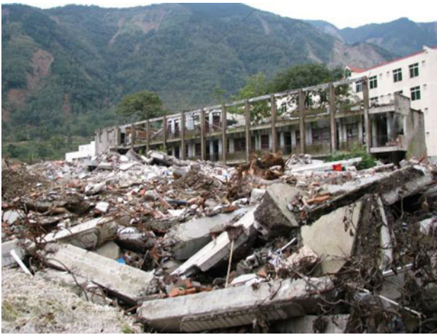
Fig. 1 Building damages at Xinbei Middle School
