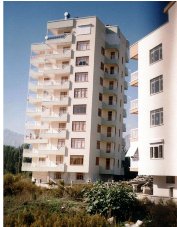
Fig. 17 Leaning structure in the study area
