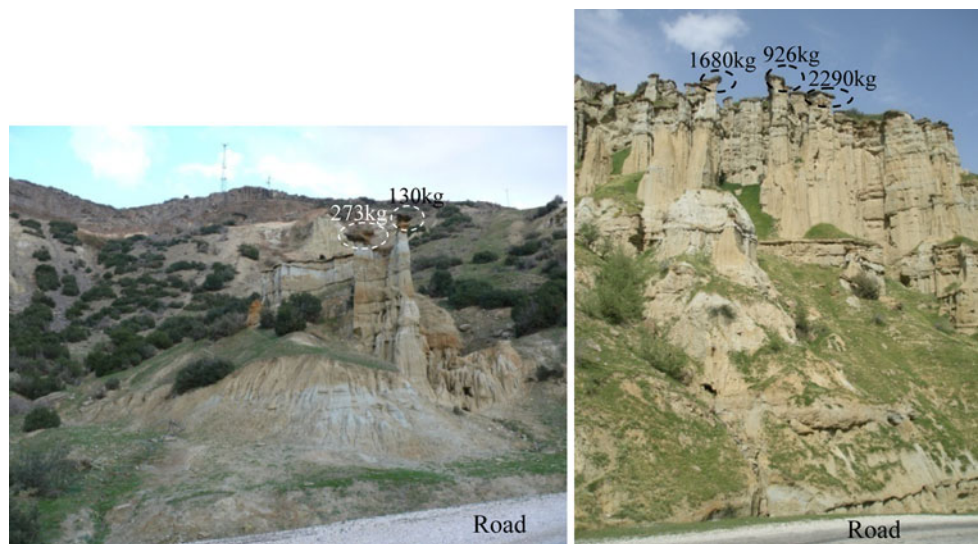
Fig. 11 Pictures of some of the hanging blocks at the top of the earth pillars
