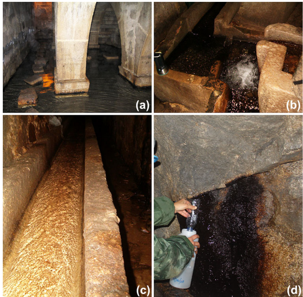
Fig. 2 Some aspects of the spring galleries catchworks: a Arca d'Água masonry reservoir (ca. XVI century); b junction of Paranhos and Salgueiros spring waters; c granitic gutter pipe; d seepage from an open sub-horizontal discontinuity
