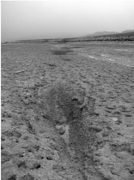
Fig. 11 Picture of the main scarp acquired in 2007. The crack was some 513 m long in May 2008. Underground water seeping into the sub-horizontal layers is responsible of this failure
