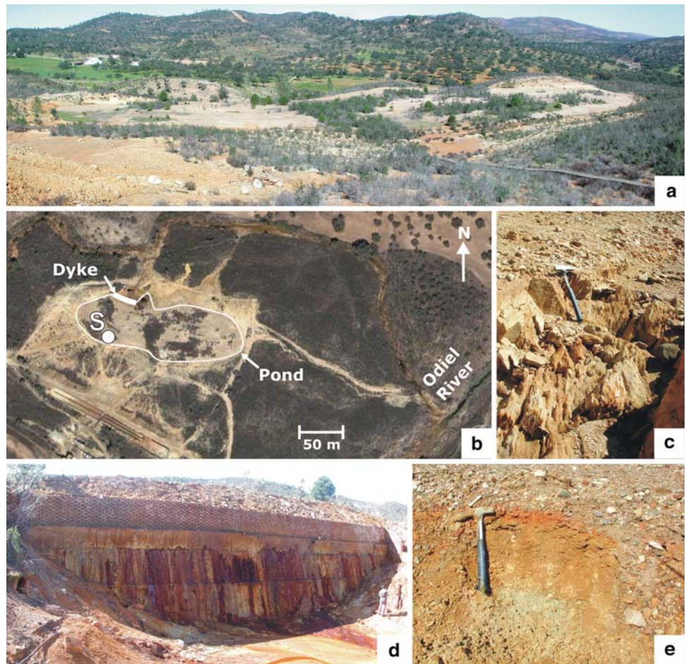
Fig. 2 a General view of the restored Mina Concepción mine pond. b Satellite image of the mine pond and its surroundings ( http://www.goolzoom.com ); the sampling location is marked as S. c Aspect of the volcanic substrate of the mine tailings, in this point covered exclusively by gravels. d Acid waters flowing through the dyke from the mine pond deposits. e Detail of the most superficial capping materials of the reclamation
