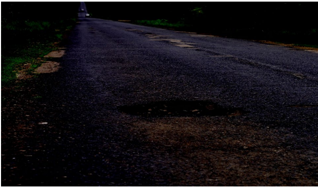
Fig. 1 Insufficient light on the road at night
