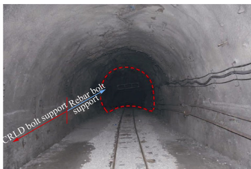
Fig. 17. Supporting effect of the CRLD bolt.
