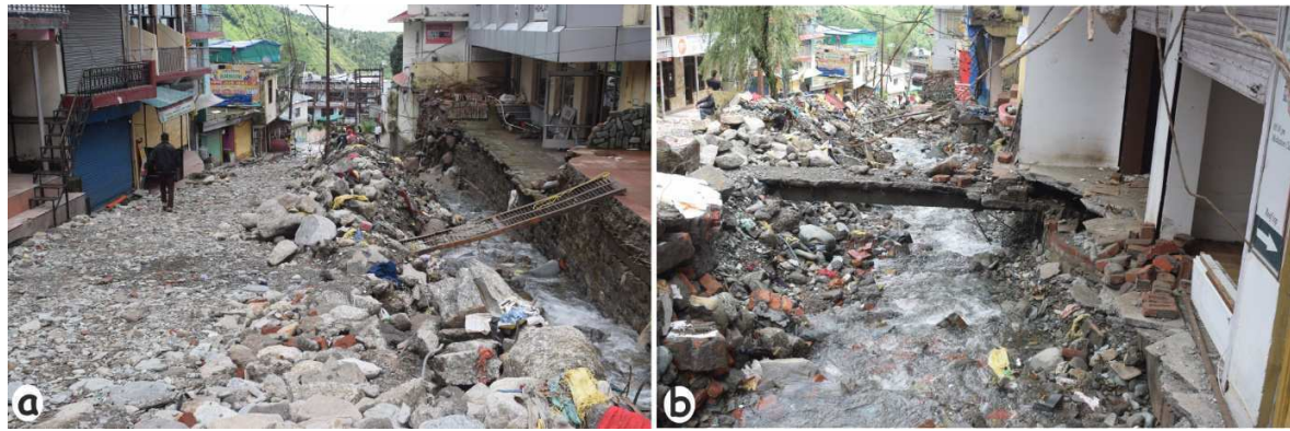
Fig.6. (a) Damage to connecting road and (b) damage to the residential and commercial establishments located by the side of the Bhagsu nala
